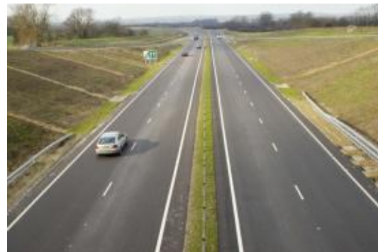
Typical Rural Open Cutting
