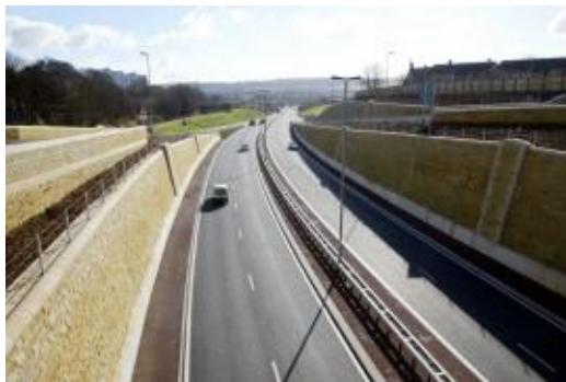
Typical Urban Retained Cutting
