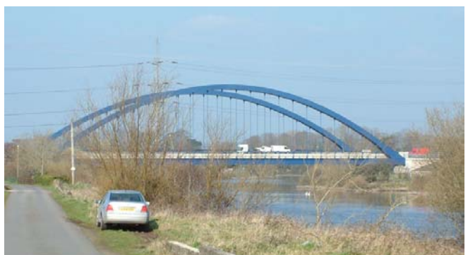
Tied Arch Bridge carrying Toome Bypass over the Lower River Bann
